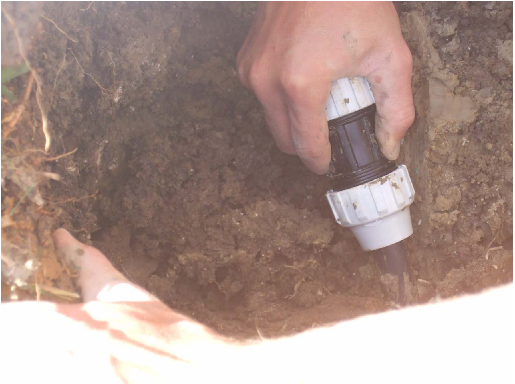
Installing FloPlast Fitting on CTS size HDPE Pipe
