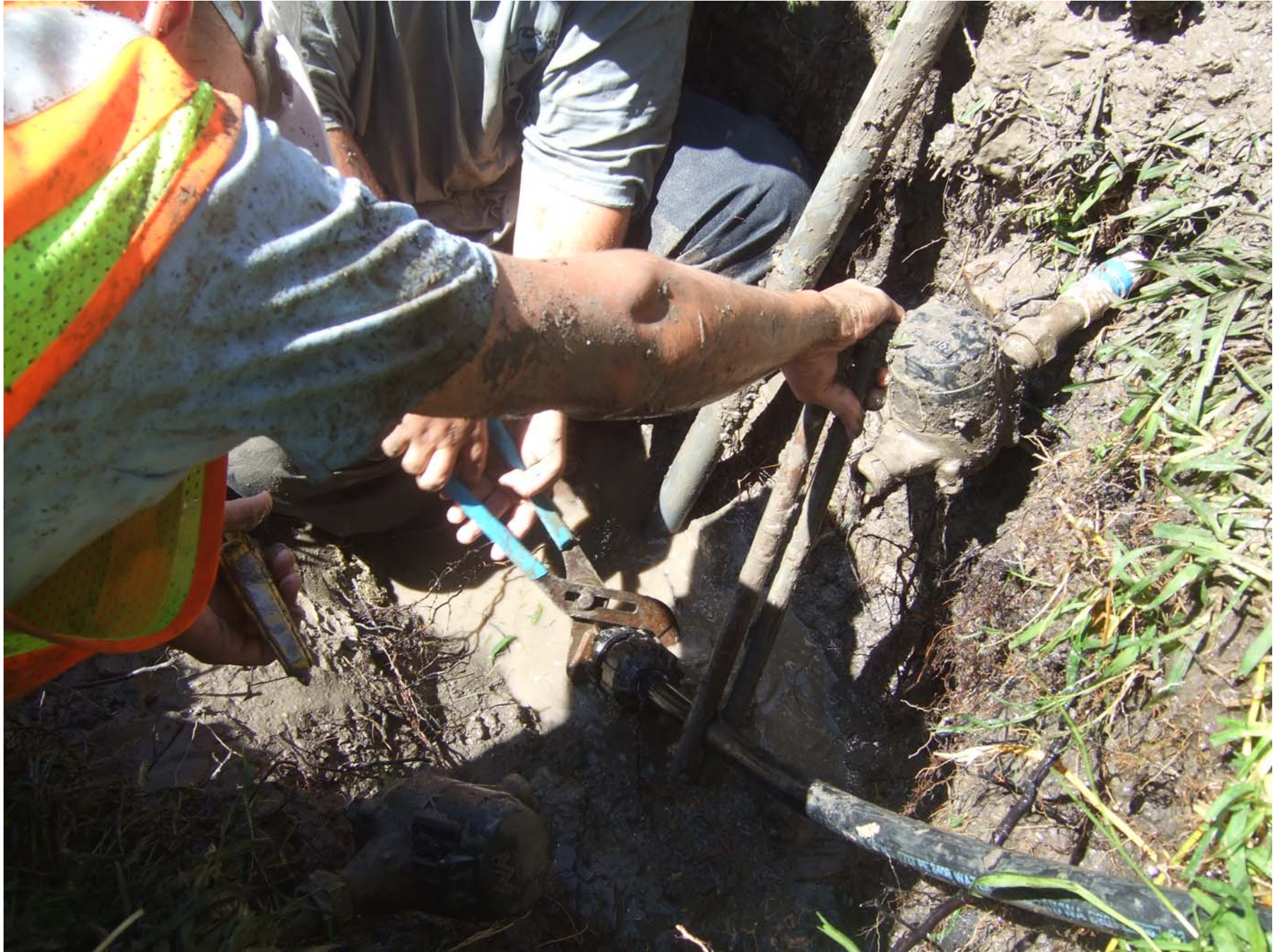
FloPlast Fitting installed—tightened down—no more running water!
