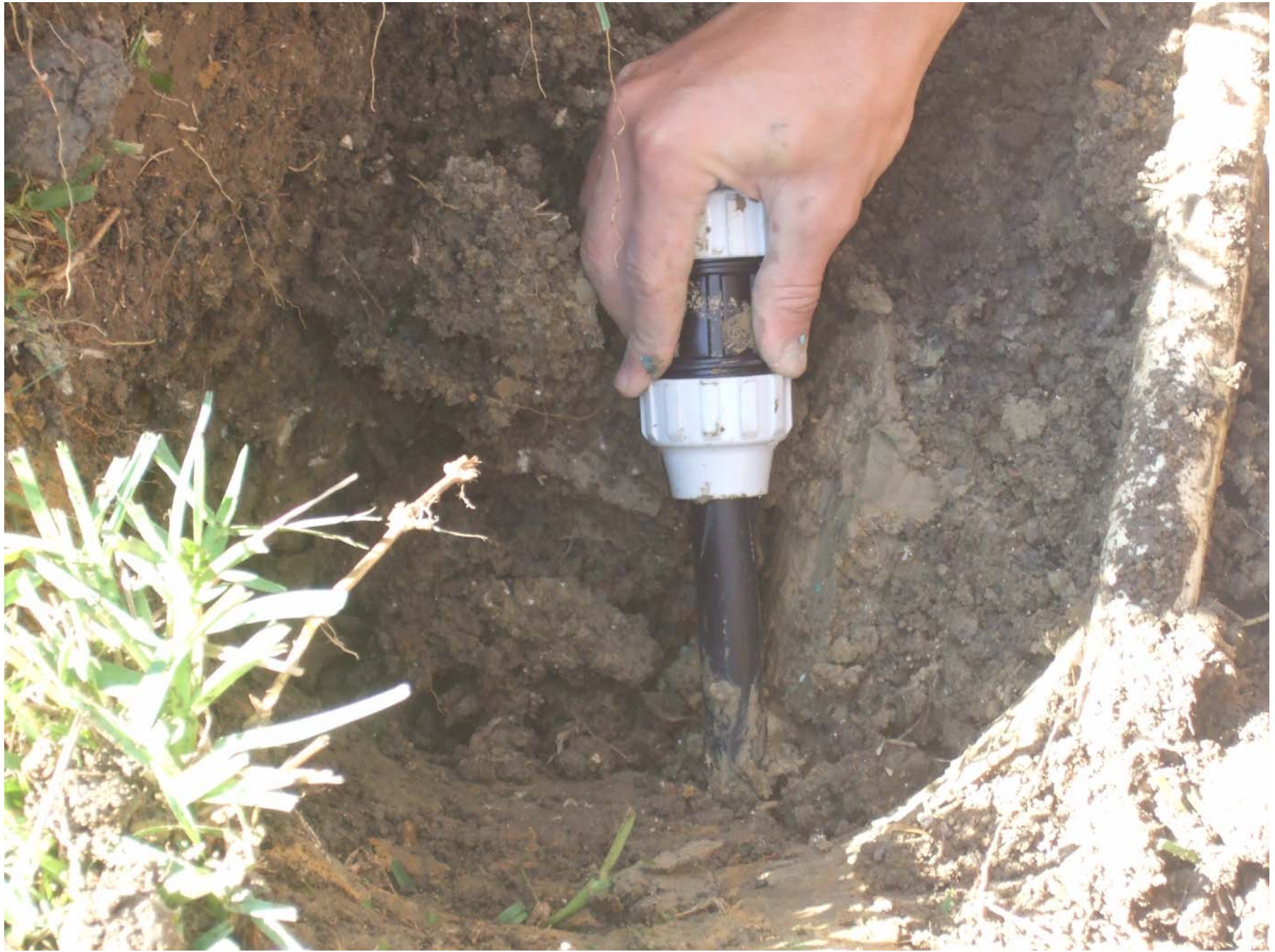
Installation as easy as—push the fitting on - click past the grip ring— click past the o'ring—tighten the nut—done!
