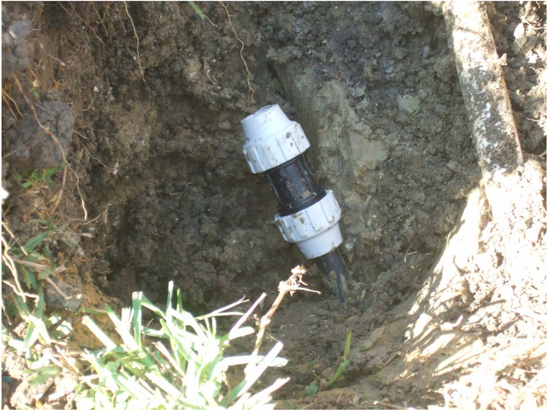
FloPlast Fitting installed—ready for the rest of the pipe
