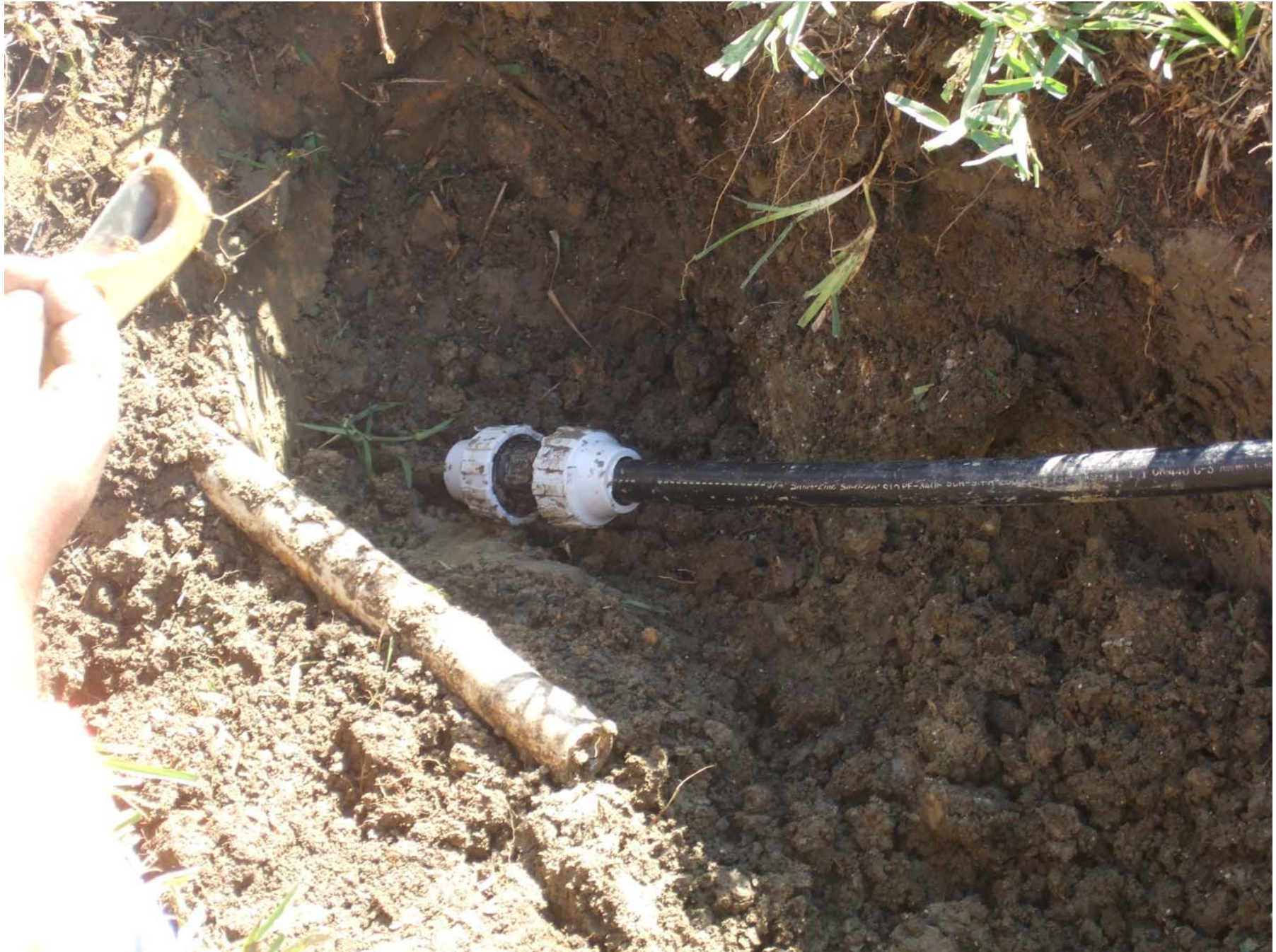
FloPlast CTS Fitting on new installation
