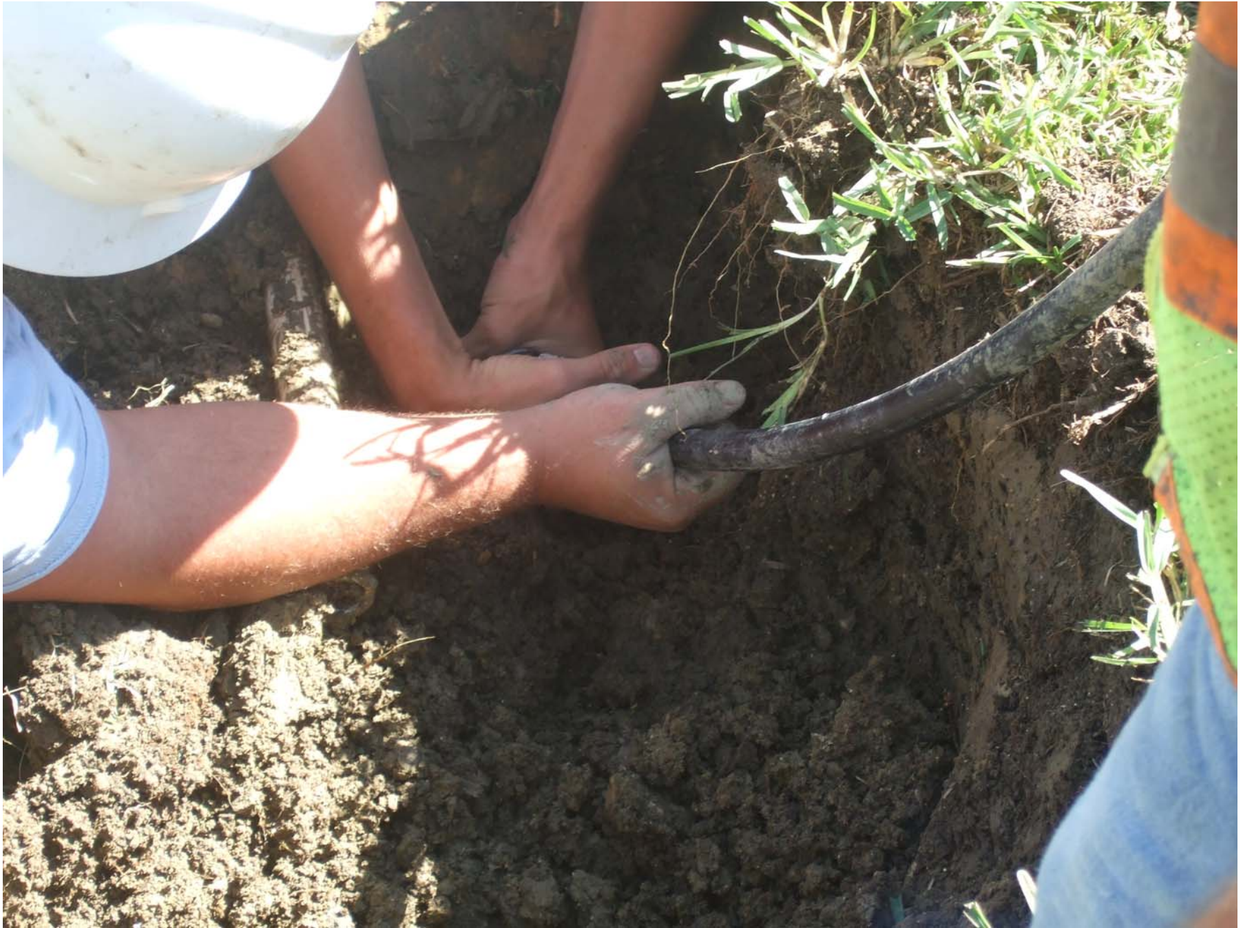
Pushing CTS HDPE pipe into new FloPlast Fitting.
